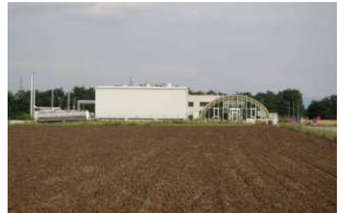
A biodiesel refinery In Germany
